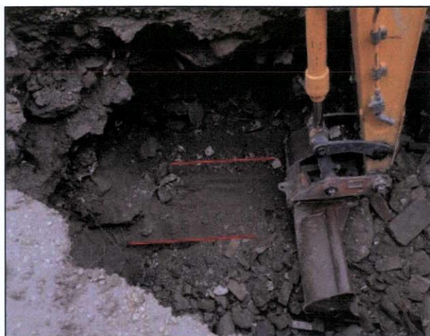
Figure 60 The structure from the north
