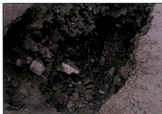
Figure 57 The floor abutting the wall foundation
