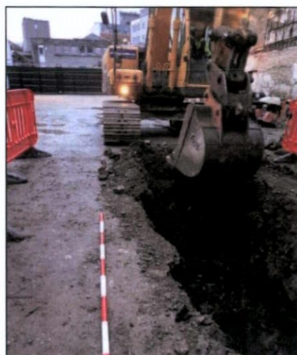
Figure 45 Trench 1, from the east
