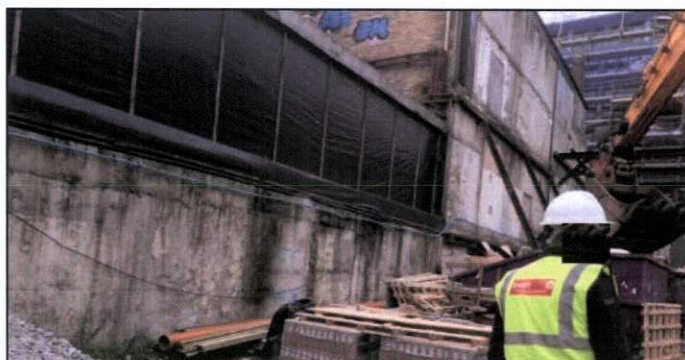
Figure 66 The south wall, west end
