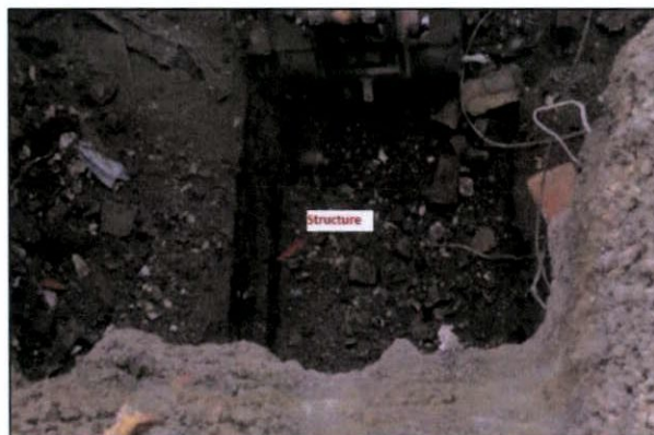
Figure 58 Foundation from the east
