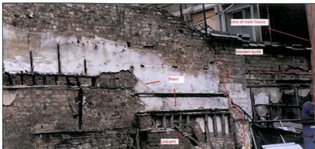
Figure 88 The stairs at the eastern end
