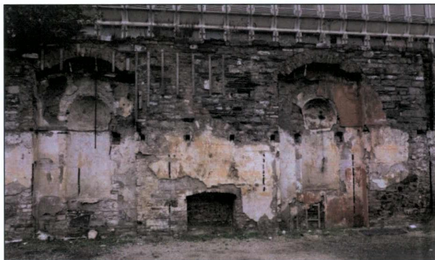
Figure 74 Building 2, from the south
