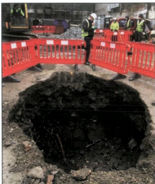
Figure 53 The expanding trench
