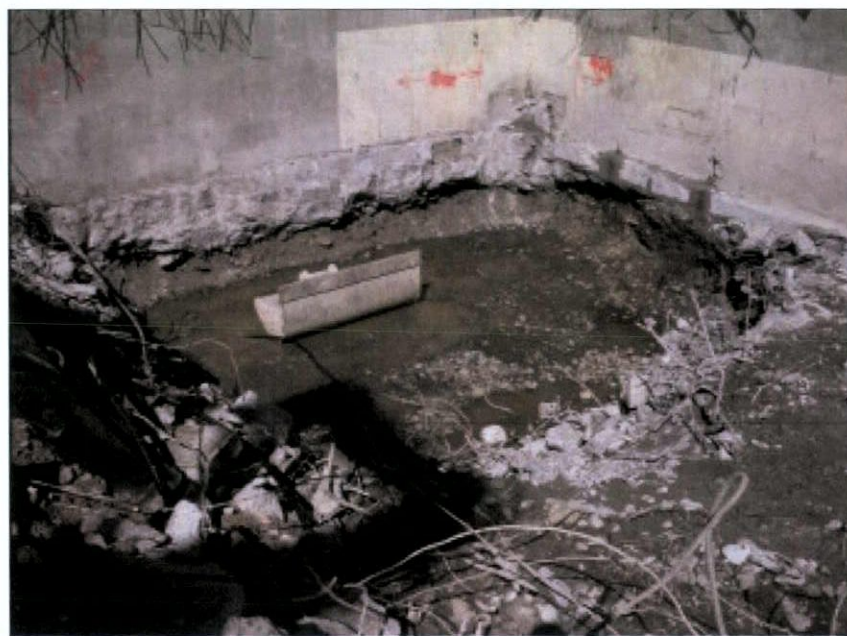
Figure 27 Trench 4, temporary crane base
