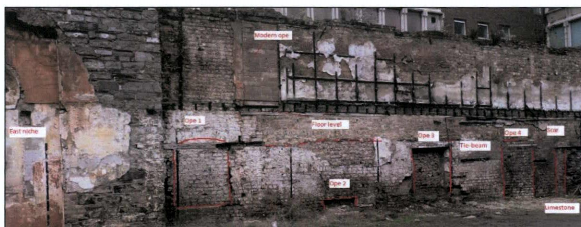
Figure 83 Building 3, from the west
