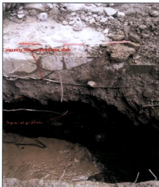
Figure 25 Trench B, concrete and natural gravels
