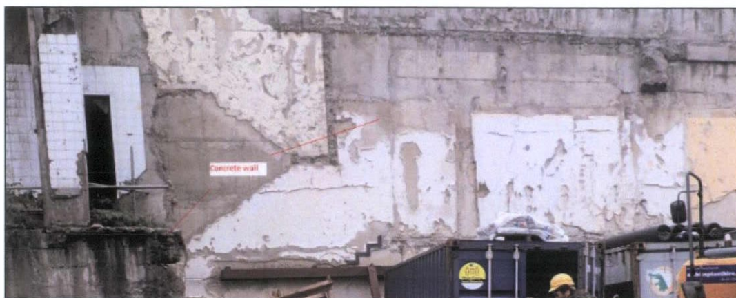
Figure 63 The north wall
